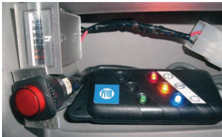
Fig. 5. View of the control panel with LED indicators. The red safety brake push button is shown by the panel, and the counter of working time of the compressors in the semi-trailer / trailer is shown above.
