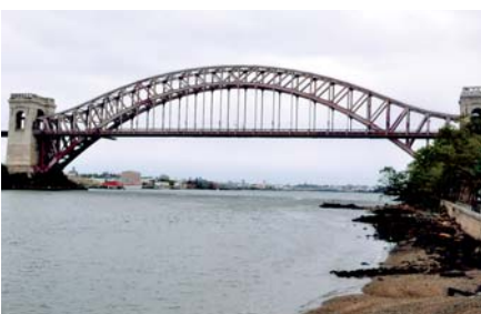
Ryc. 38. Gustav Lindenthal, Hell Gate Bridge w Nowym Jorku, 1916, l_{\text{max}} = 298,0 \text{ m} [3]
