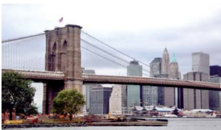
Ryc. 36. John i Washington Roeblingowie, Brooklyn Bridge w Nowym Jorku, 1869–1883, l_{\text{max}} = 486,0 \text{ m} [3]
