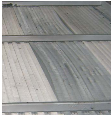
Figure 2. The buckled tube bundle.
