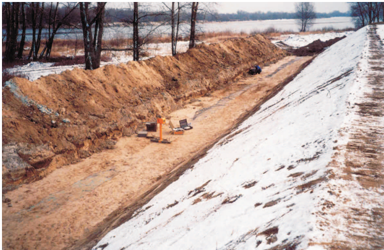
Fig. 4. View of the experimental section
