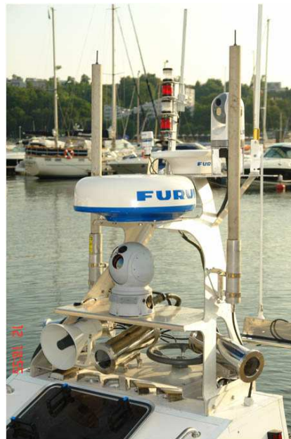
Fig. 3. Placement of navigational devices and communication system aerials on the mast.
