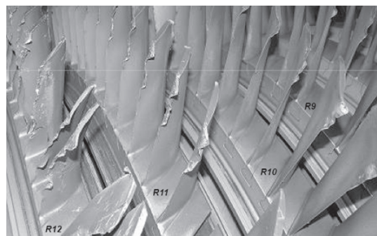
Fig. 3. Compressor moving blade damage
