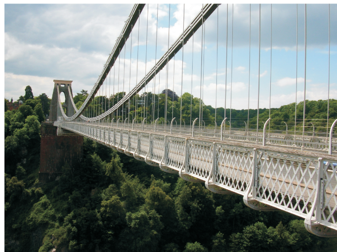
Fot. 44. Clifton Suspension Bridge I.K. Brunela w Bristolu z 1864 r.
