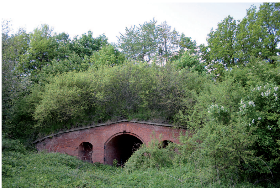
Fig. 12. The shed shelter surrounded by lush invasive greenery (photo by A. Trepka)
