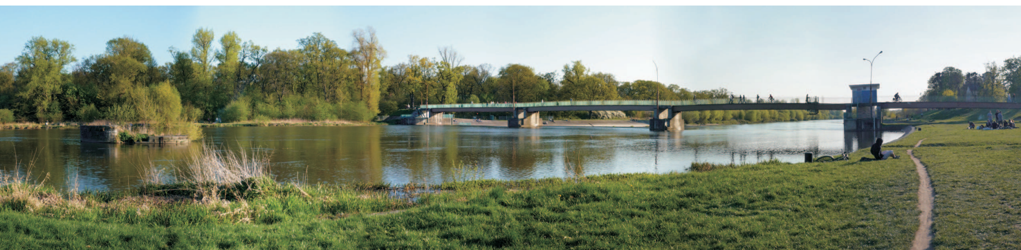
Fig. 3. View of barrage Opatowice
