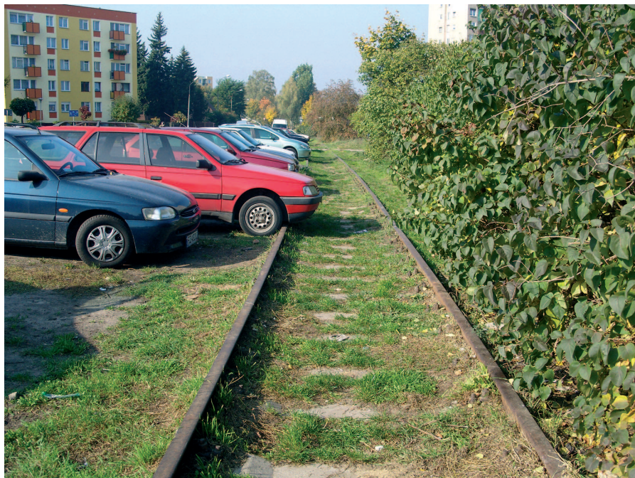
Fig. 6. The abandoned railway line connecting Zielona Góra and Koźuchów
