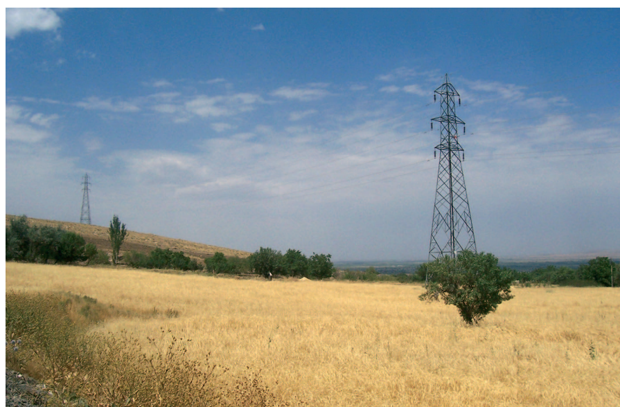
Fig. 8. New infrastructures created new rural landscapes in relationship with the agricultural fields
