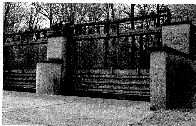
Flood sluiceway in the Lipki-Oława Polder dike
