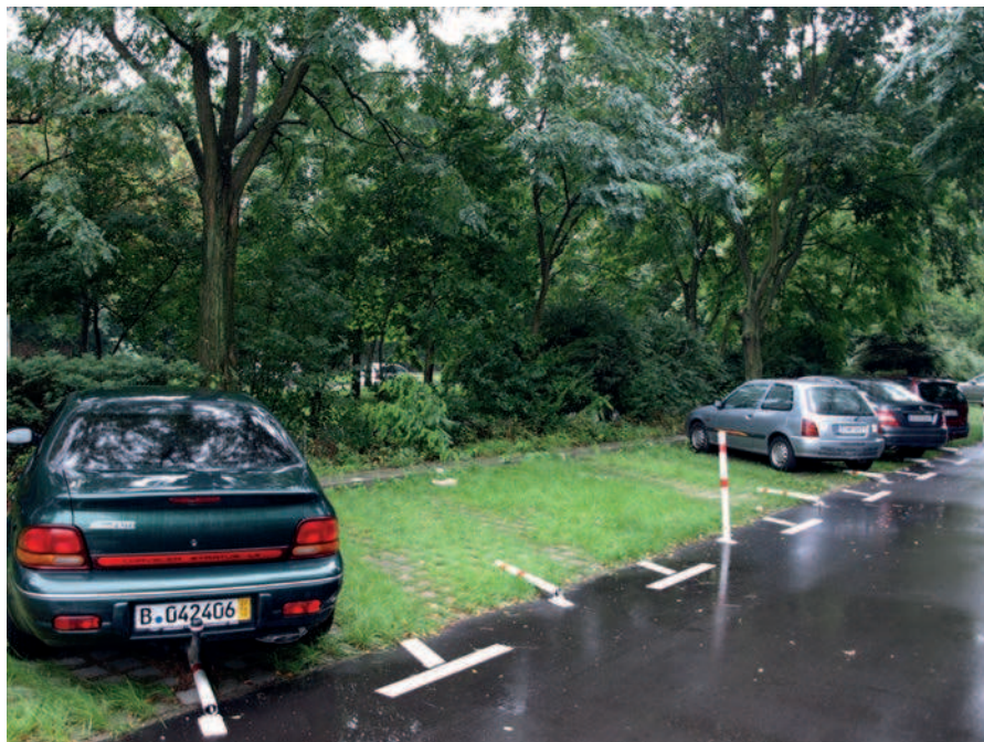
Fig. 3. Ecological surface made of green joints on the parking places (photo by J. Burdziński)
