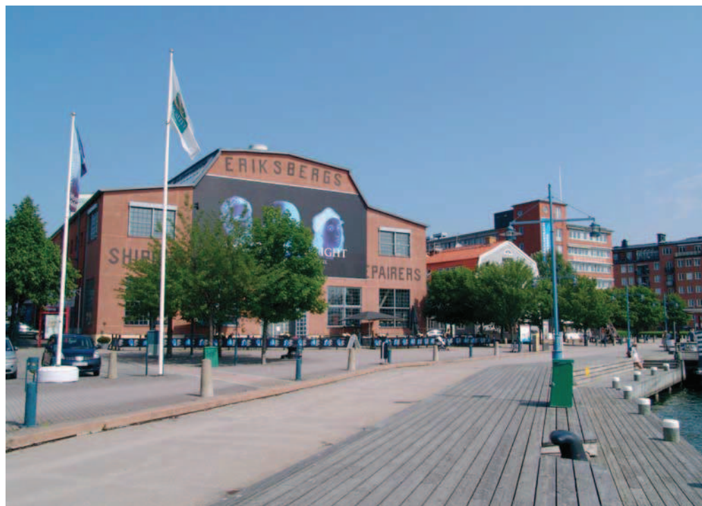
Fig. 6. A node of a public realm network – square within a quay promenade, arranged in front of former shipyard workshops, preserved and adapted for public uses
