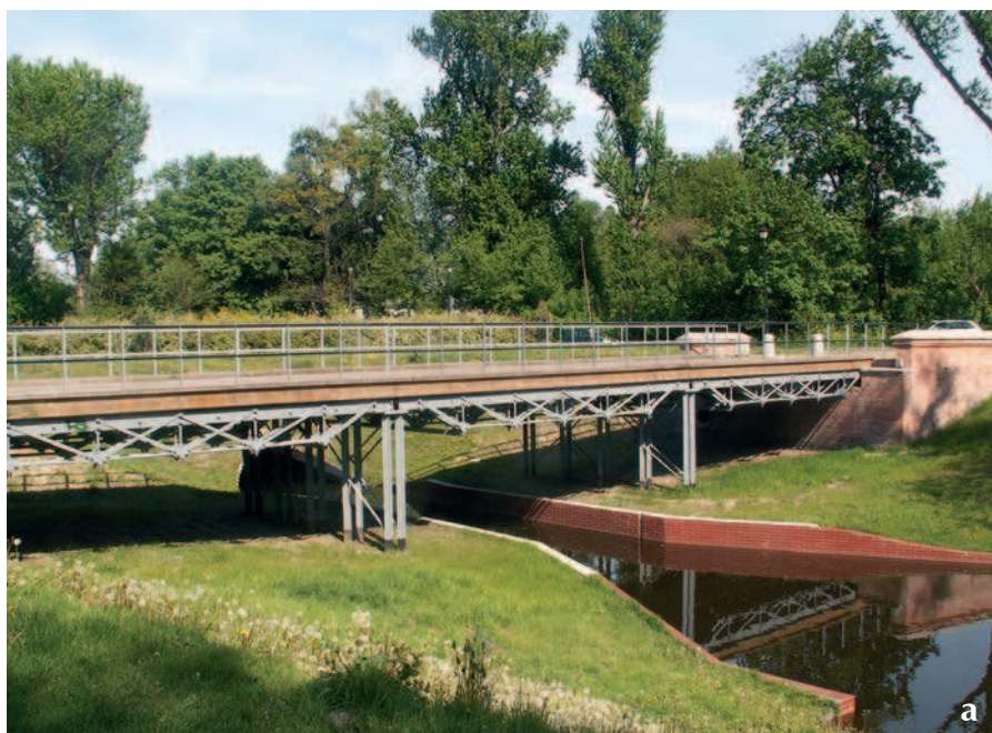
Fig. 1. a. Historical bridge after reconstruction, b. New bridge
