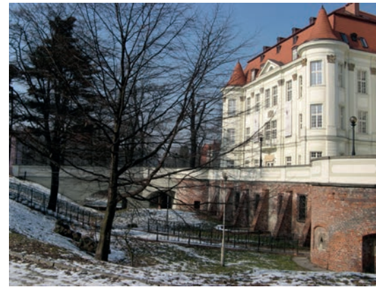
Fig. 5. View of palace in Leśnica
