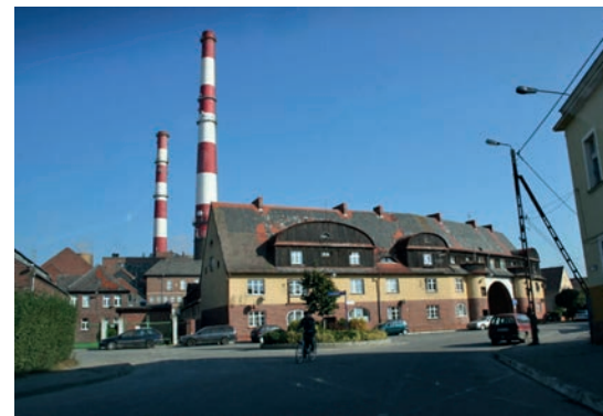
Fig. 14. View of the steelwork in Siechnice
