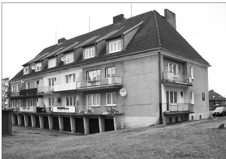
Fig. 1. The analyzed building
