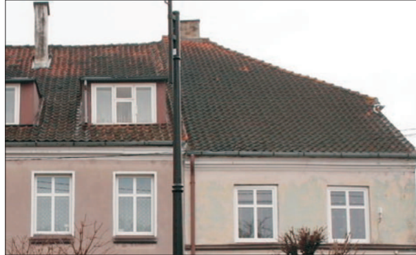
Fig. 9. A mansard roof
