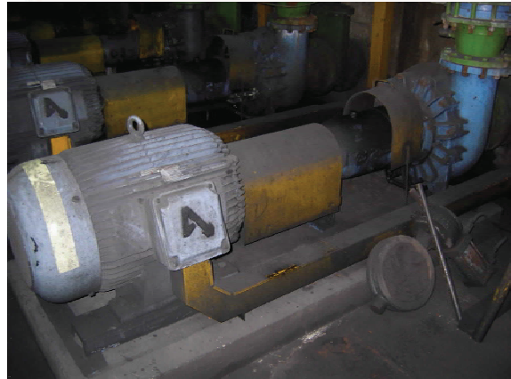
Fig. 6. Measurement points in a motor-pump
