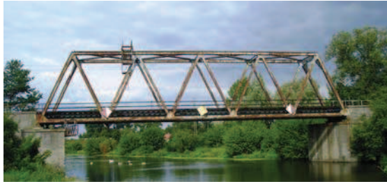
Fig. 1. Railway truss bridge monitored in Nieporet
