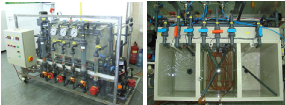
Fig. 1. Pilot membrane installation equipped with MF/UF and NF/RO membranes
