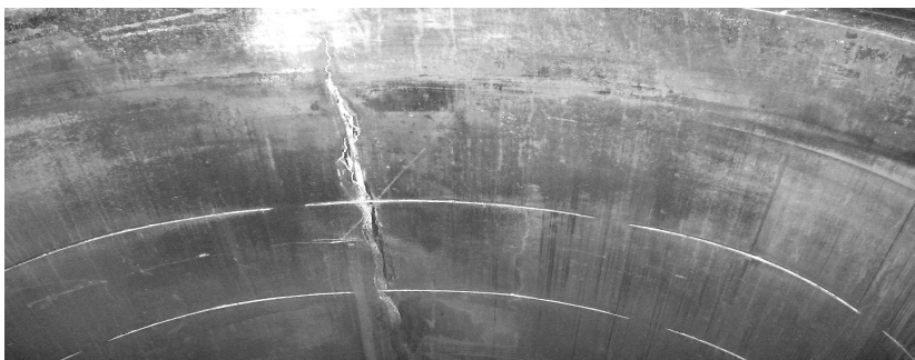
Fig. 6. Crack of the cylinder liner in the area of lubricating grooves
