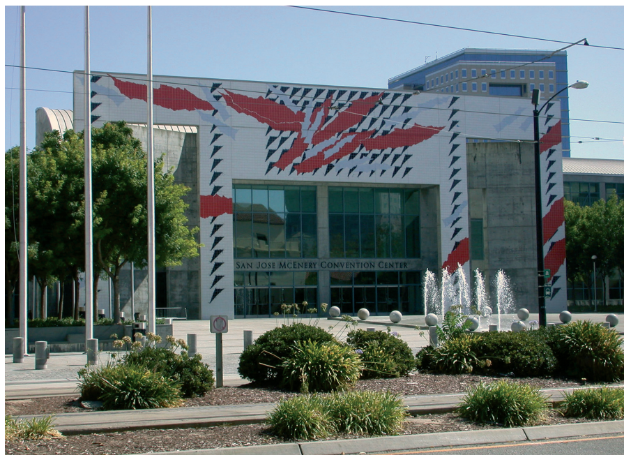
San Jose Convention Centre, arch. Mitchell/Giurgola, 1989 Fot. M. Bąkowska
