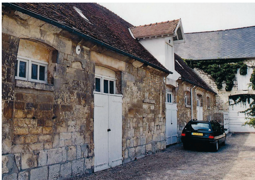
Post inn in Gournay-sur-Aronde – view inner yard and facilities
