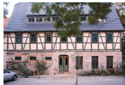
The regional building, ground floor – stone masonry, first floor – brick naggged timber wall
