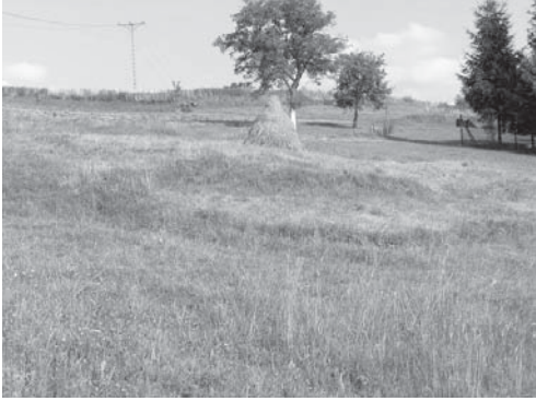
Fig. 8. The crown of the landslide and its deformation and soil ripples, with characteristic steps, hollows and interstices, which are the result of the colluvial masses movement in the western part of the landslide near Skawinska street. (Photo by A. Borecka)
