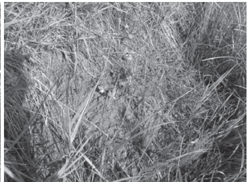
Fig. 7. Water seeps from the crown of the landslide in its western part near Skawinska street. (Photo by A. Borecka)
