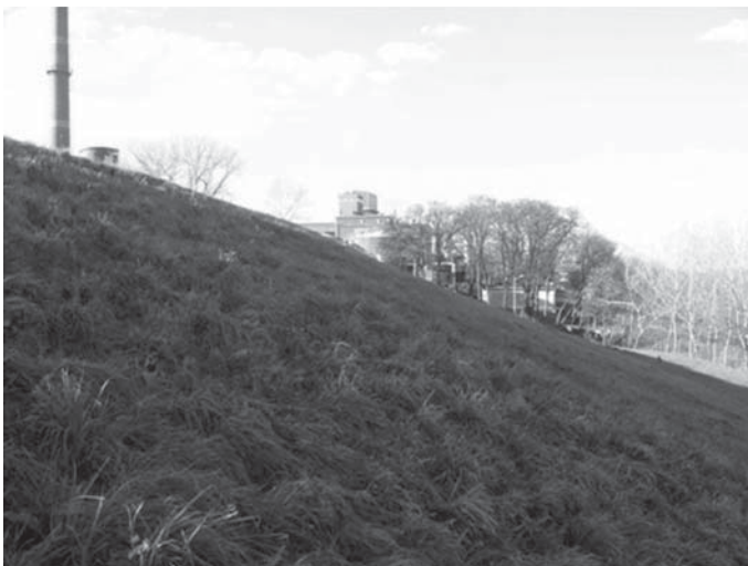
Fig. 1. Present view of the embankment dam [5]
