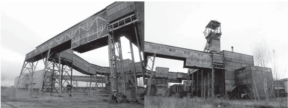
Fig. 7. Coal reloading bridges. Pithead Andrzej III with hoisting tower on the right. Photo A. Zaborska-Jagiełło 2009
