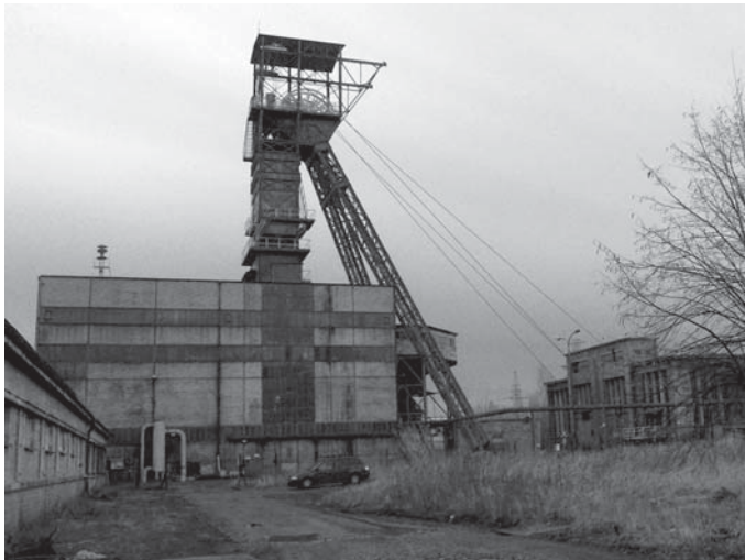
Fig. 9. Pithead Andrzej III with hoisting tower. Part of guildhall on the left. Engine hall on the right. Photo A. Zaborska-Jagiello 2009
