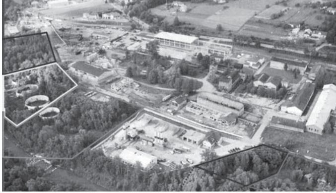
Fig. 12. Sowliny, view of industrial area of the refinery — west view — concrete factory — on the north cylindrical refractory walls — on the background historical buildings — oils hall, fire station. Photo Limanowa County, offer of the plots for sale 2011
