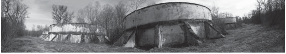
Fig. 9. Sowliny, tubular, refractory walls made with brick, west view. Photo A. Szewczyk 2011
