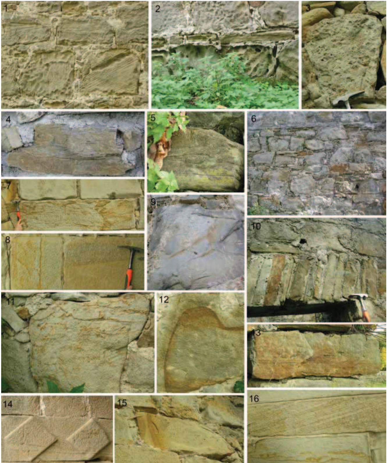
sandstone (g) with convolute lamination; 6 – part of wall built of coarse-grained sandstones with parallel lamination in places (i) and fine-grained, tabular sandstones with parallel and cross lamination (i, g); 7 – water-escape sedimentary structures within coarse-grained sandstone (i); 8 – sharp boundary between coarse-grained and medium-grained sandstone (i); 9 – flute-casts (good indicators of paleocurrents directions) on a bottom surface of sandstone layer (g); 10 – “briquettes” from darker, brownish, fine-grained sandstones (g) and lighter, tabular, coarse-grained sandstones (i) in stone door-frame; 11 – water-escape structures within coarse-grained sandstone (i); 12 – coarse-grained sandstone with single grains of glauconite (?g); 13 – coarse-grained massive sandstone passing to fine-grained up top of layer (g) – part of layer in overturn position (top turned down and bottom turn up); 14 – decorative ornamentation of stone door-frame made of coarse-grained sandstone with cross-lamination (i); 15 – coarse-grained sandstone (i); 16 – cross-laminated and massive coarse-grained sandstone (i).
