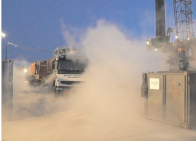
Fig. 3. Preparation of foam cement with N_2
