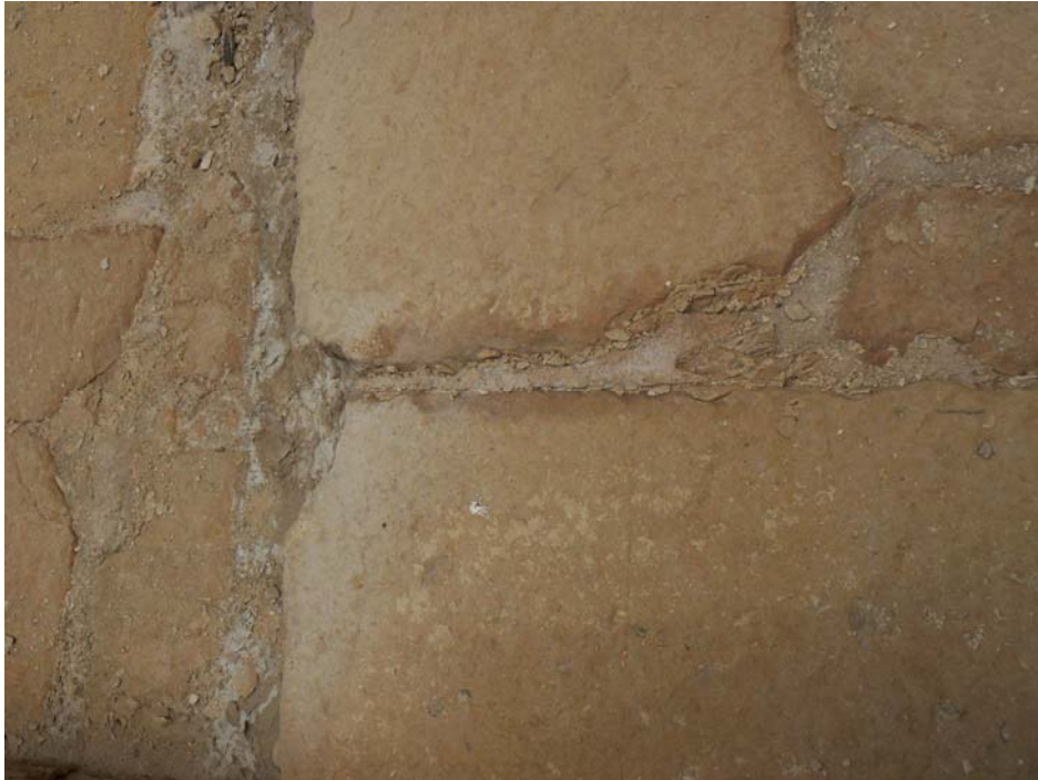
Photo 4 Light, fine crystallized gypsum at species between blocks used as material cementing blocks of Abu Rowash Pyramid
