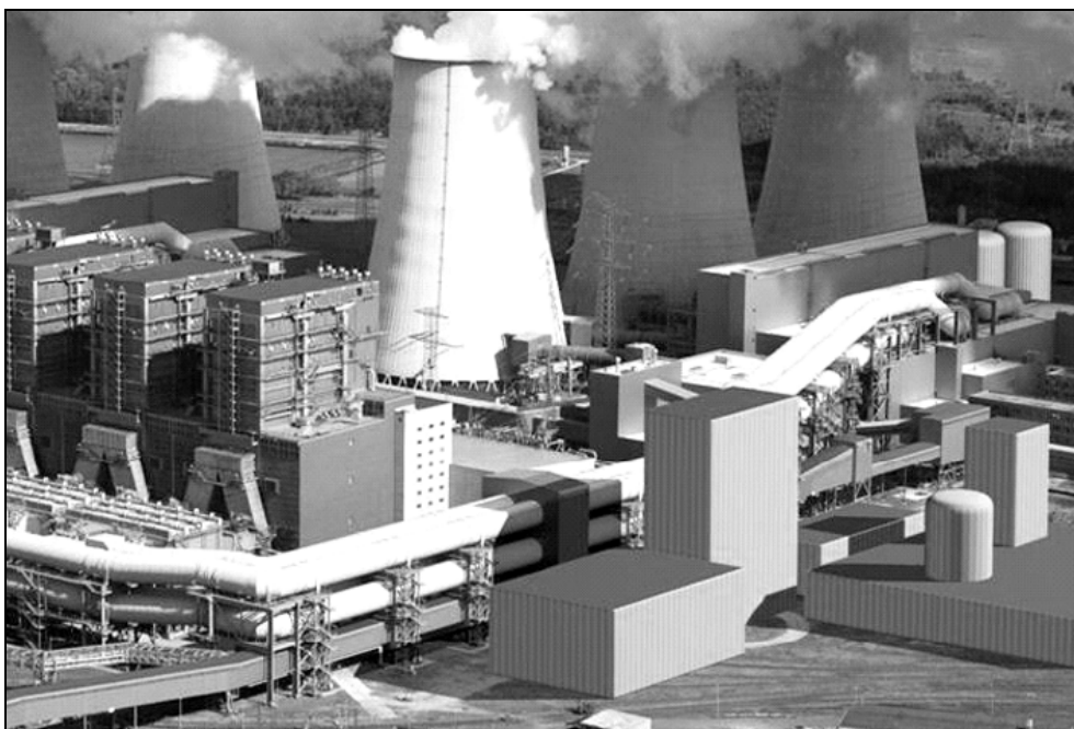
Fig. 6. Demonstration plant in Jämschwalde
