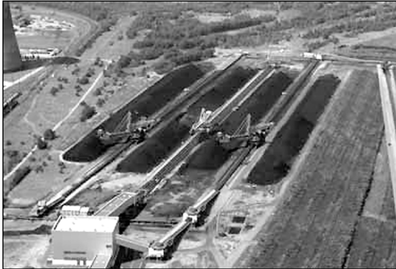
Fig. 1. Target configuration of the Boxberg coal stockyard in 2010
