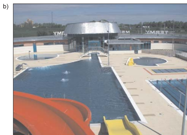
Fig. 1. Absorption heat pump (Sanyo, 2.7 MW) cooperating with high-temperature boiler (Viessman, 1.9 MW) in Mszczonów geothermal plant (a). The thermal pool “Termy Mszczonów” located near the plant (b)
