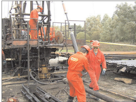
Fig. 9. “Gas Gun” propellant stimulation tool ready to be run into Well L (Tab. 3)
