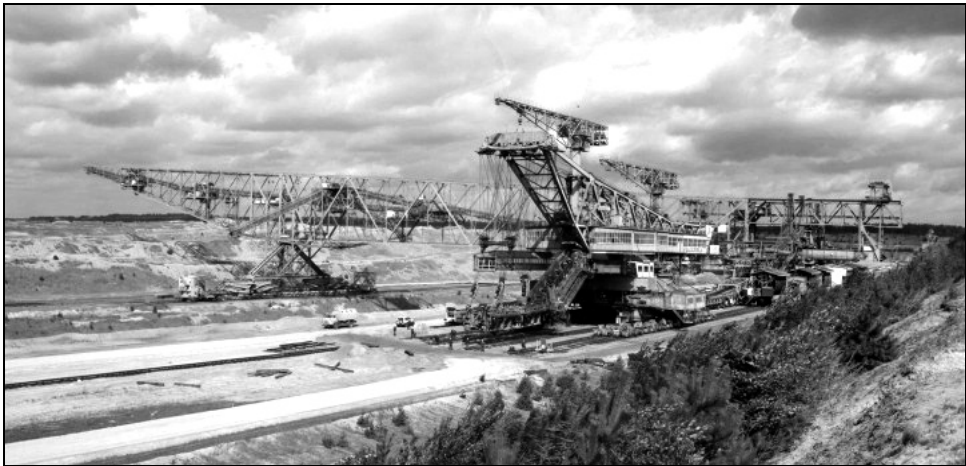
Fig. 4. Refurbishment of the overburden conveyor bridge F60 in the Reichwalde mine
