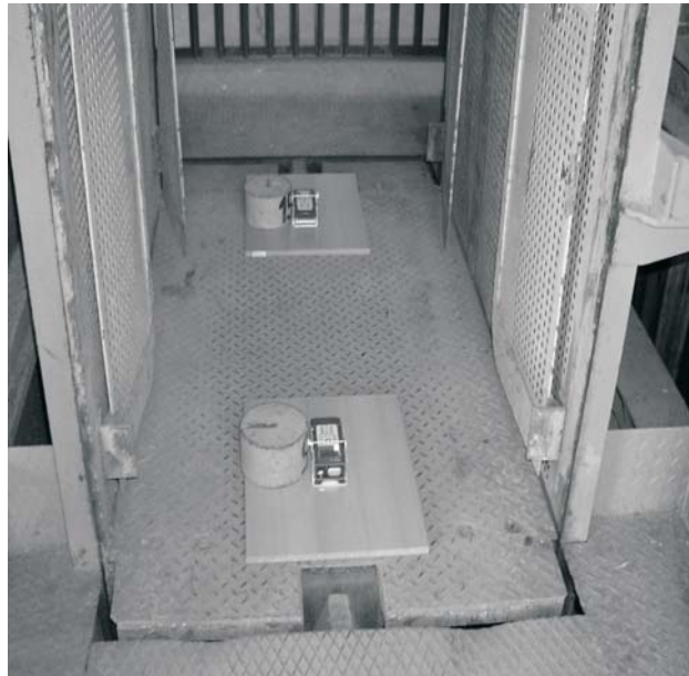
Fig. 1. Measurements of guide frontal spacing using DISTO plus laser distancemeters in the shaft Campi in the Bochnia Salt Mine
