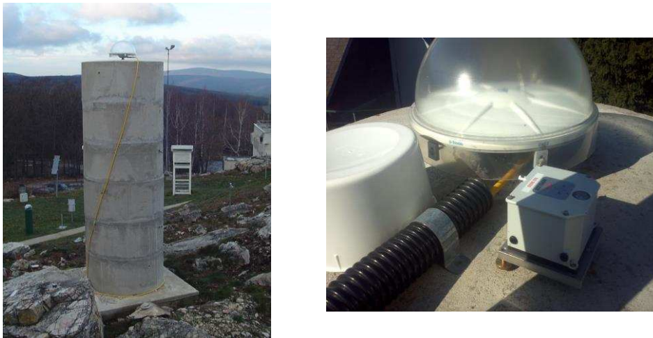
Fig. 1. Pillar monument at station Modra-Piesok MOP2 (left) and detail with GNSS antenna and inclination sensor (right).
