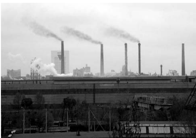
Fig. 1. View on the plant before implementation of resource-conserving technologies
