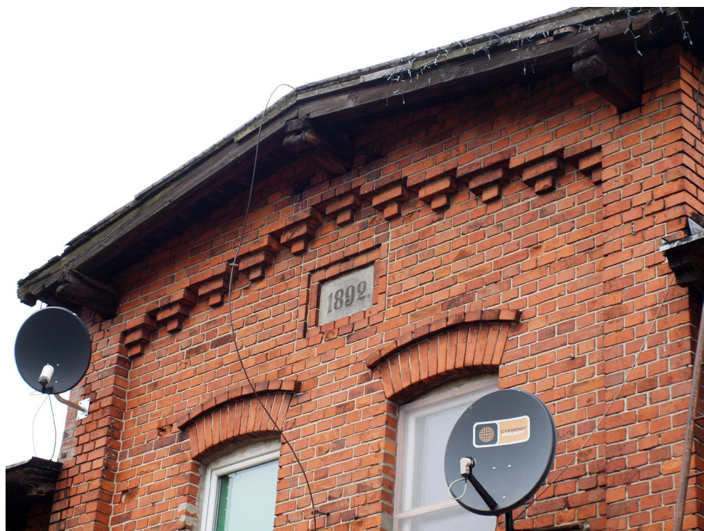
Fig. 2. Anielin, an example of brick architectural detail
