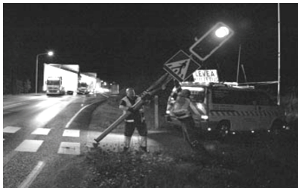
Fig. 8. Preparation of the route to pass a wide load.
