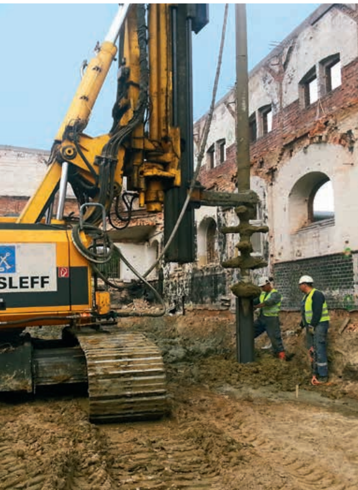
Palisada z kolumn DSM, fot. Aarsleff Sp. z o.o.
