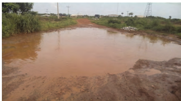
Photo 3. Water logged environment as result of lack of drainage system (phot. O.A. Lawal-Adebowale)
