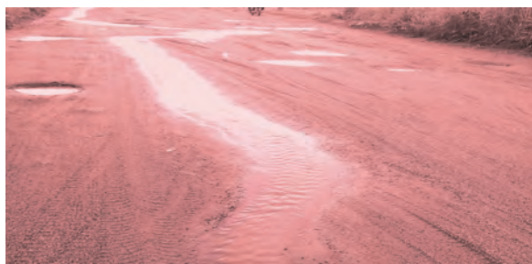
Photo 2. Scattered multiple water pores and temporary stream along the road (phot. O.A. Lawal-Adebowale)
