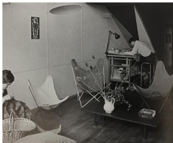
Fig. 12. Interior of a typical residential unit, 1952; Source: Cohen J.L., 2008.
