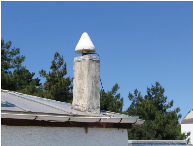
Fig. 1 TRAB GNSS Reference Station
