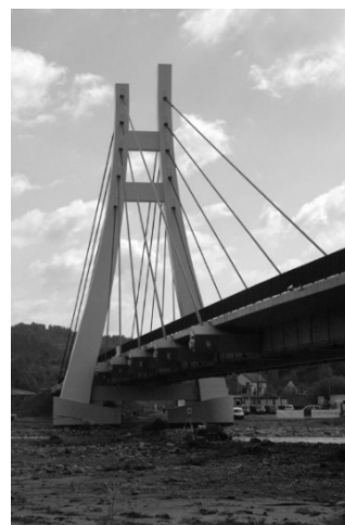
Fig. 1. Suspended cable-stayed bridge in Zembrzyce Rys. 1. Podwieszony most w Zembrzycach
