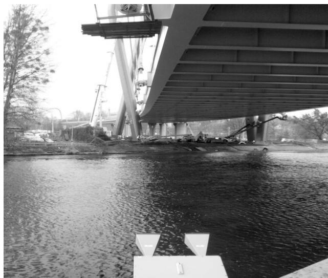
Fig. 4. Measurement of the main bridge span in Bydgoszcz
