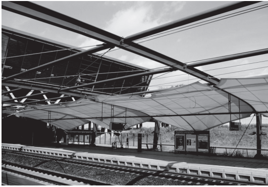
Fig. 16. Leipzig/Halle Airport Railway Station, platform hall, source: own work
