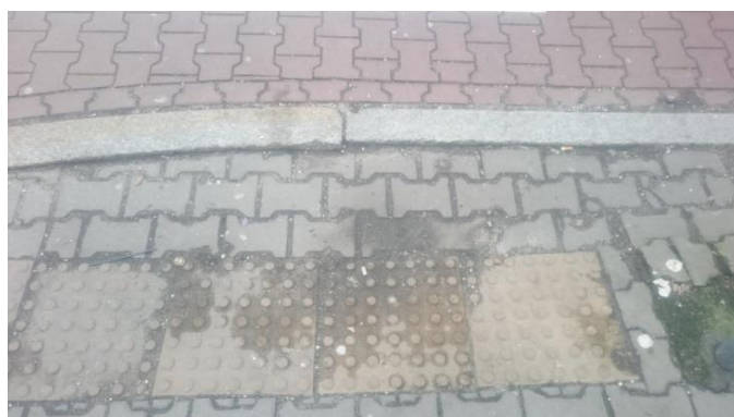
Fig. 6. Tram stop at Bernardyński Square. Yellow warning paint is nearly totally invisible and warning texture is worn out (2018). Own elaboration
