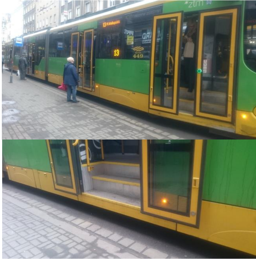
Fig. 10. East side of Gwarna street. Stop is maladjusted to the requirements of the user; lack of markings of the edge with yellow paint, lack of warming tabs for blind people, lack of elevation enabling ergonomic use of low-floor trams as well as the use of them by people on wheelchairs (2018). Own elaboration
