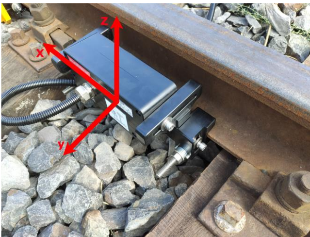
Fig. 1. Rail-mounted measuring antenna with the indicated directions of the plane
